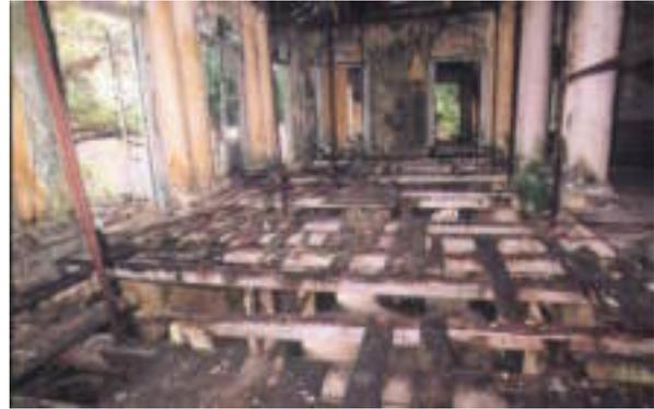
Figure 4. The damage floorboard
