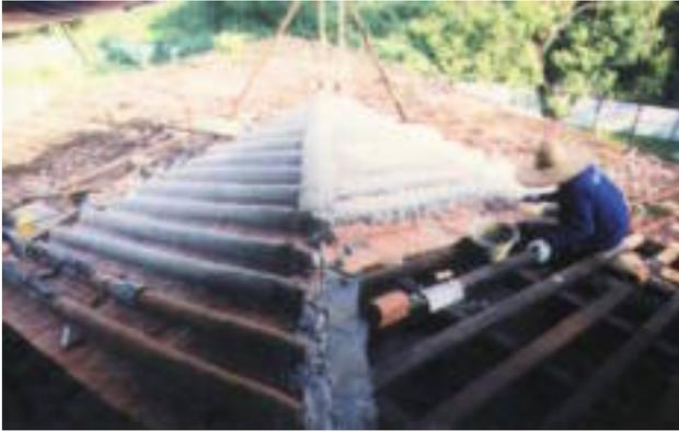
Figure 10. Laying and fixing new roof tiles
