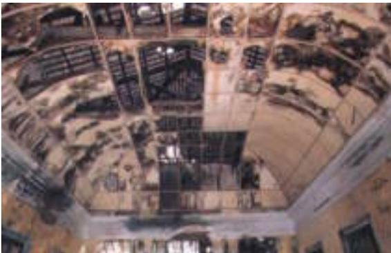
Figure 3. Ceiling board was damaged cause by water penetration through leaking roof.
