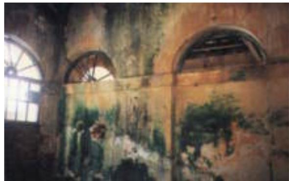
Figure 5. Wall surface covered with fungal and mosses.
