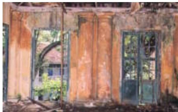
Figure 6. The upstairs building condition, timber door was rotten and damage. The columns were mostly effected with rising damp and crumbling plaster problems.
