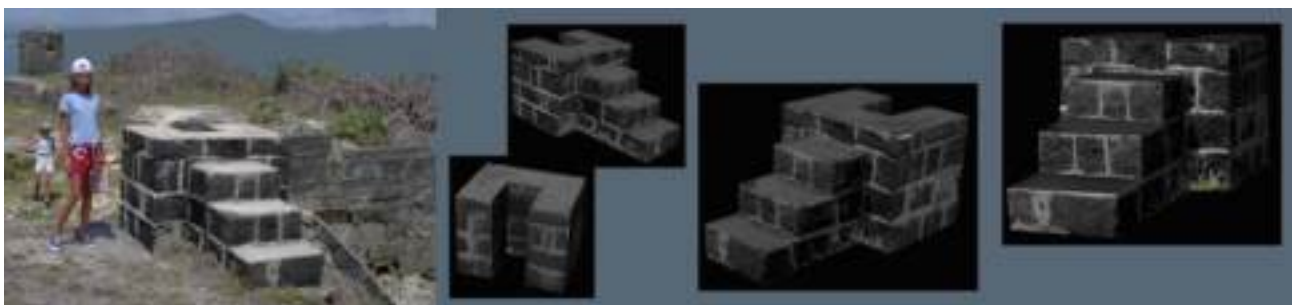
Figure 8. The small stepped structure, probably a flag pole emplacement, on Ile de la Passe, Mauritius, was reproduced as a 3D model in PhotoModeler by Çağatay Kariptaş. The cropped portion of photograph used for each flat plane was matched to the corresponding surface of the model.
